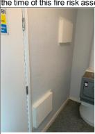
As recommended at the time of the previous fire risk assessment, the air bricks between the electrical room and bin chute room on the seventh floor have been appropriately fire stopped.
