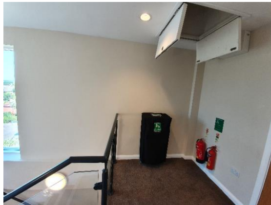
Roof hatches inspected
